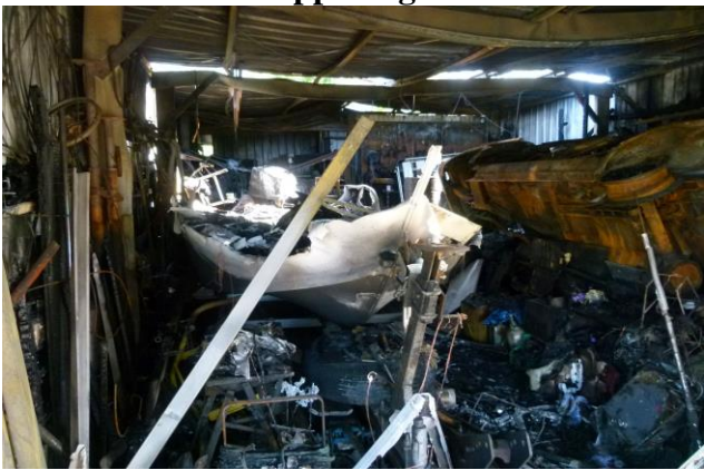
After the fire NB 8"angle iron beam behind boat bent
